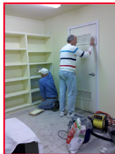
Jim Carey and Frank Roehrig paint the new library.
